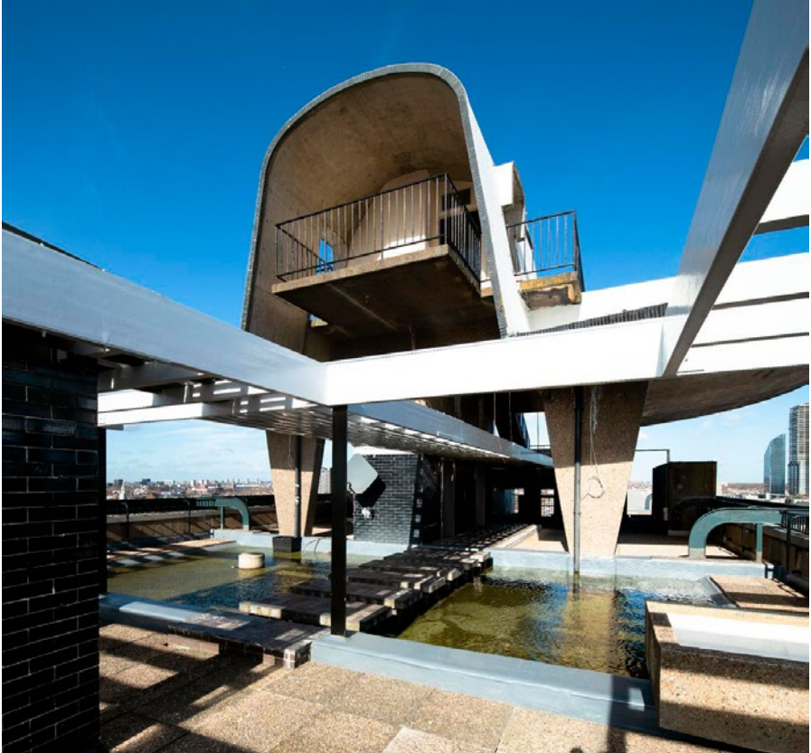
Great Arthur House rooftop as part of The Golden Lane Estate in London, designed by Chamberlin Powell and Bon in the 1950s. (Historic England Archive)
